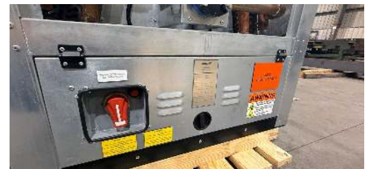
SERVICE / ACCESS VIEW Power, controls, and disconnect access
